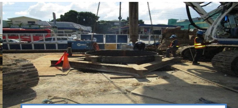
Positioning of steel casing @ Doña Carmen
