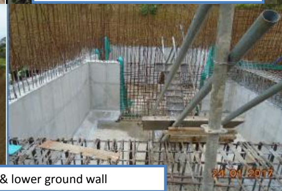
Completed Iron pouring concrete
