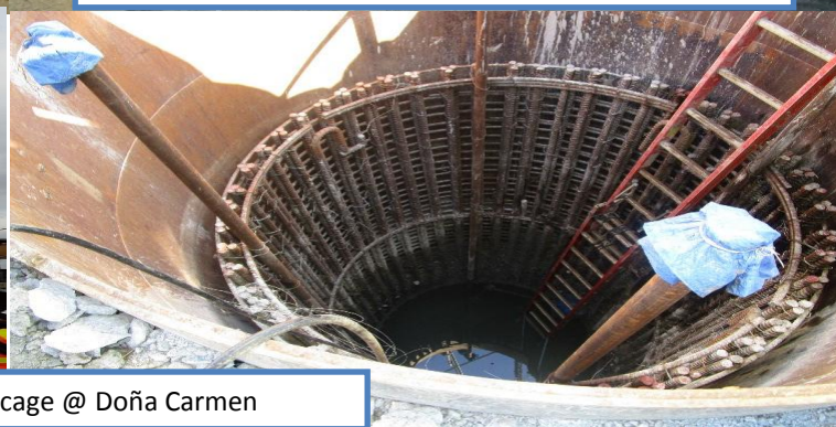
Positioning of steel casing @ Doña Carmen
