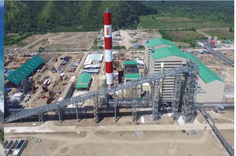
LIMAY 2X150MW POWER PLANT
