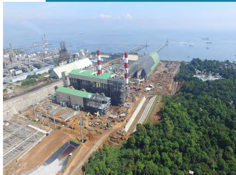
LIMAY 4X150MW POWER PLANT
