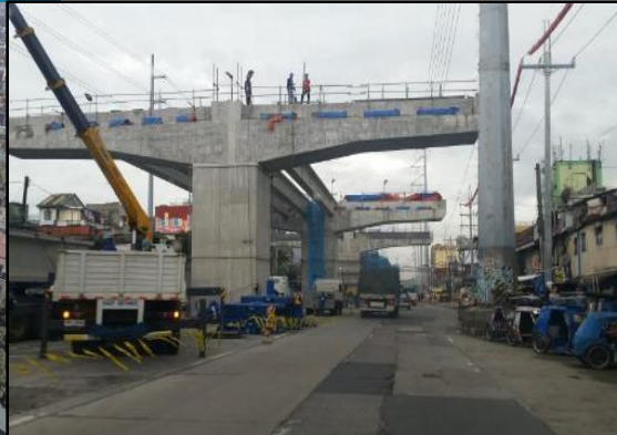
Ongoing works on Section 3
