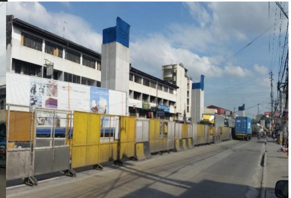
Ongoing works on Section 4
