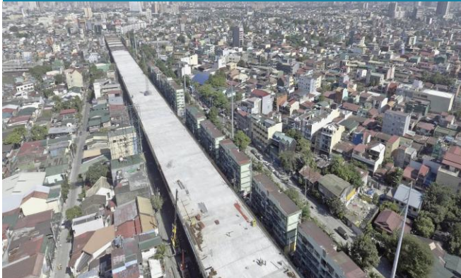
Ongoing works on Section 1
